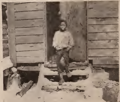
The Condition in Which We Find Them.
